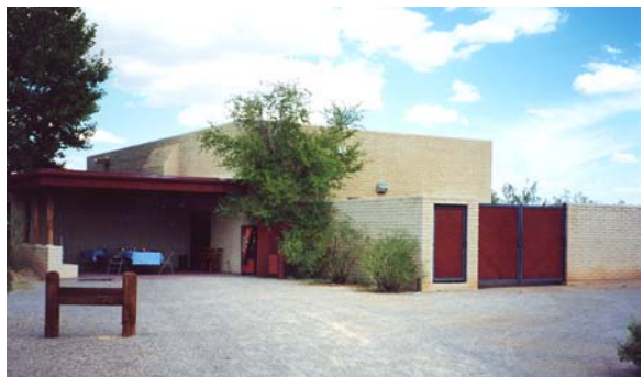
Visitor Center - Rear View
