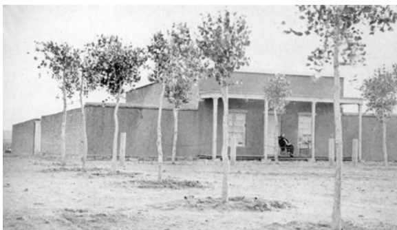
Figure A5.25. The single dwelling at the west side of the row of officers' quarters, photographed by Nicholas Brown in July 1867. Courtesy of Museum of New Mexico, Negative No. 55044. Note the structure and yard wall are stuccoed on the front only.
